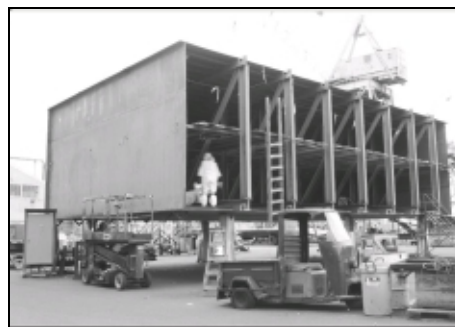
Digital image of fabricated dry-dock wing wall (Courtesy Todd Pacific Shipyards)
